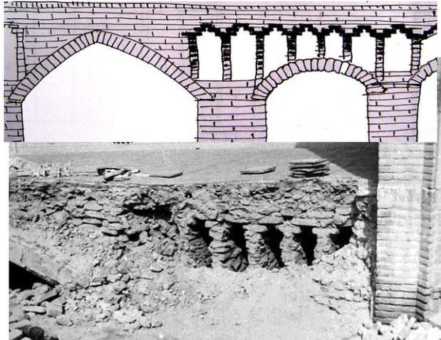
**Figure 9: picture and chart of caisson-making on vault of cellar in Borujerdis' House, Kashan.**
