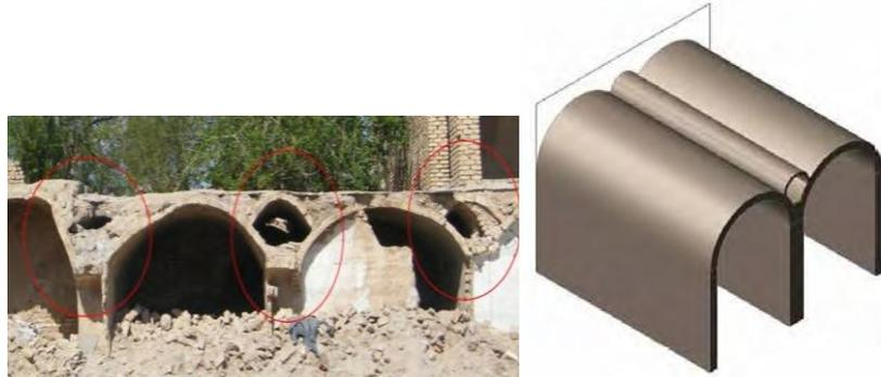
**Figure 3: Two vaults close together and the caisson-making between them.**
